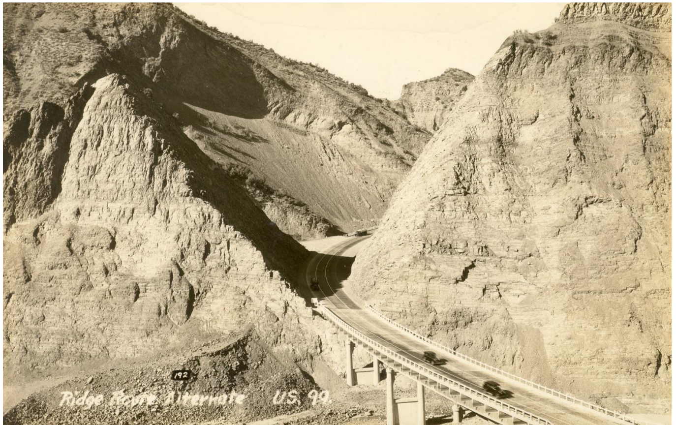
Pyramid Rock and Cut along the Ridge Route Alternate
