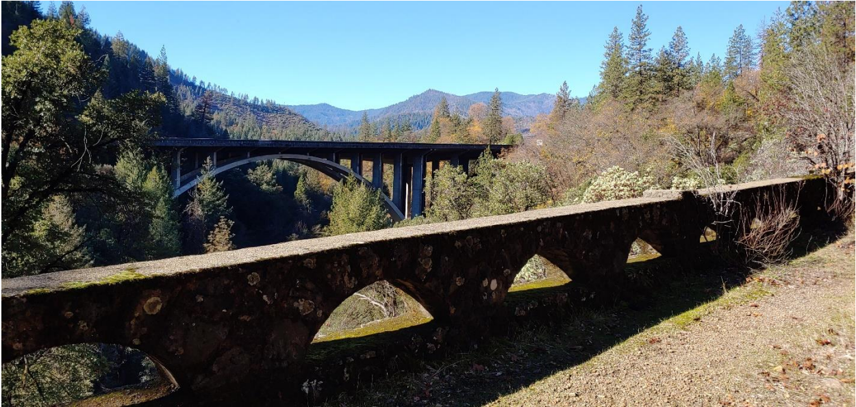
Looking toward the “new” 1956 (widened in 1989) bridge on I-5
