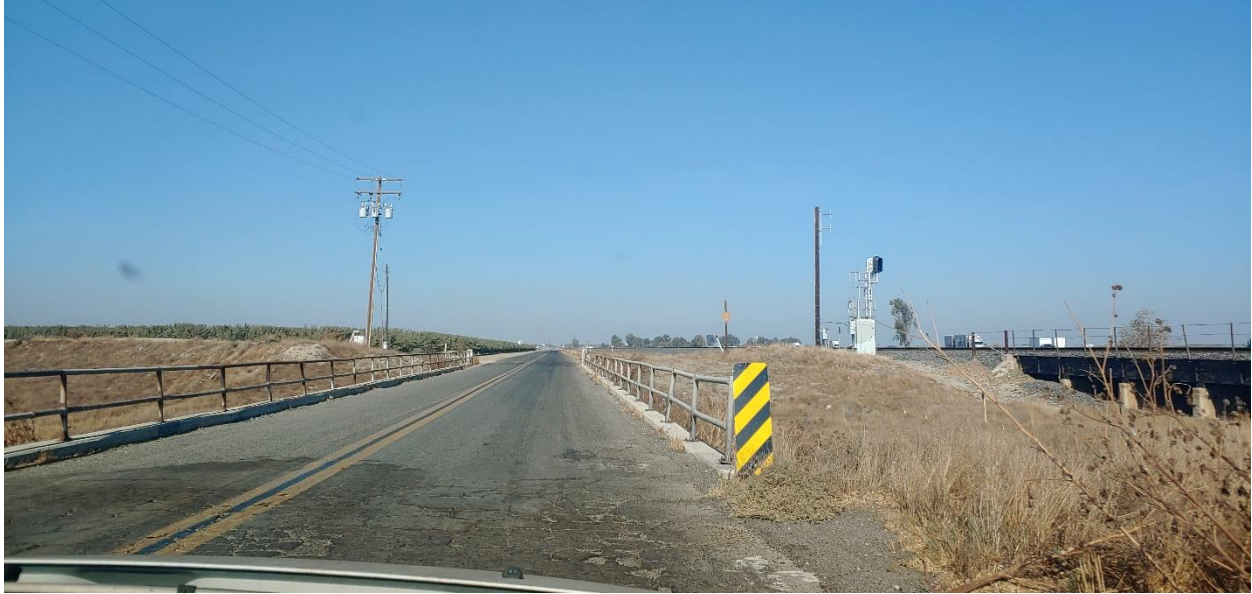
South Branch Tule River Bridge (46C-0004) from 1917
