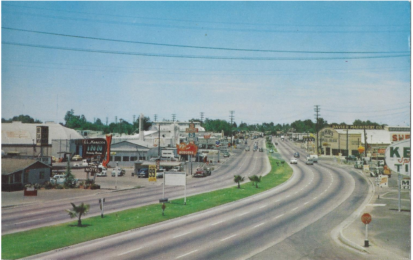
Golden State Avenue looking north from 23rd St / Junction US 466
