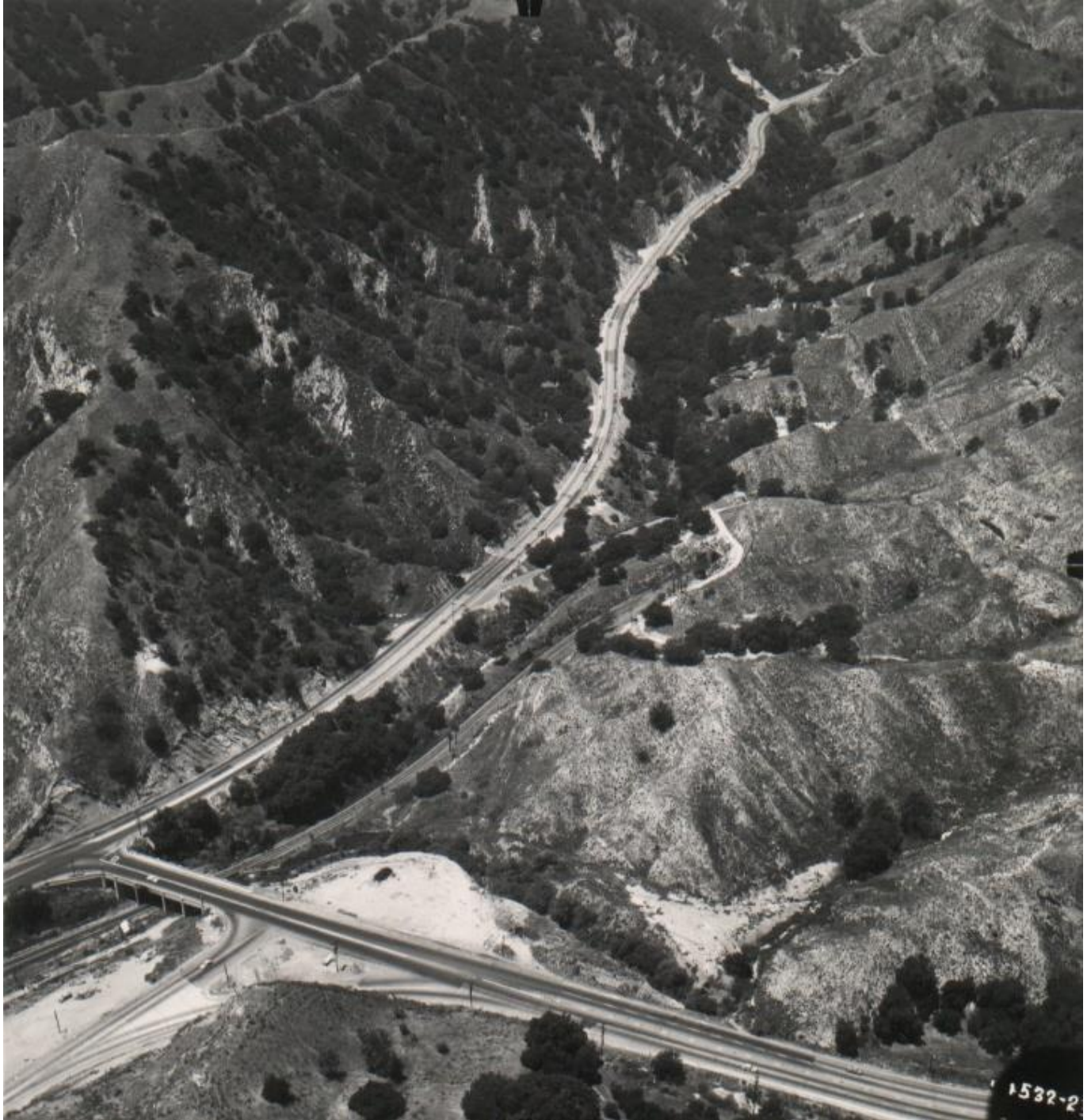
Looking north through Weldon Canyon in 1949. Courtesy – Caltrans.
