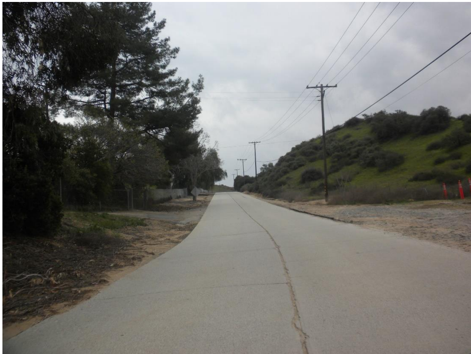
1925 Concrete section near Calimesa (Roberts Road)
